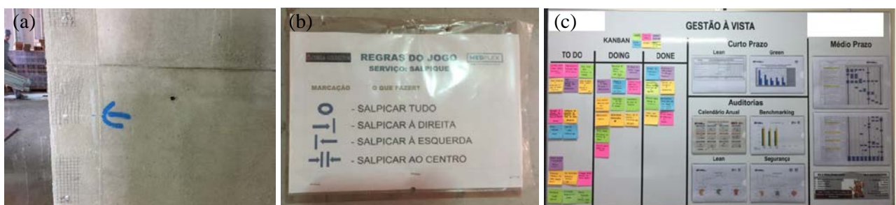
Figure 5: Example of VM best practices identified: (a) (b) Spray marking of the kind of roughcast and its explanatory sheet (Company A), and (c) Visual performance and planning boards (Company B)
