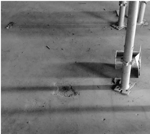
Figure 1: Floor concrete holes requiring patching work
