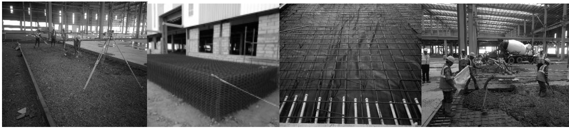
Figure 2: (a) Surface Levelling, (b) Reinforcement Mesh prepared in advanced, (c) LDPE Sheet and Reinforcement Mesh., (d) Concreting
