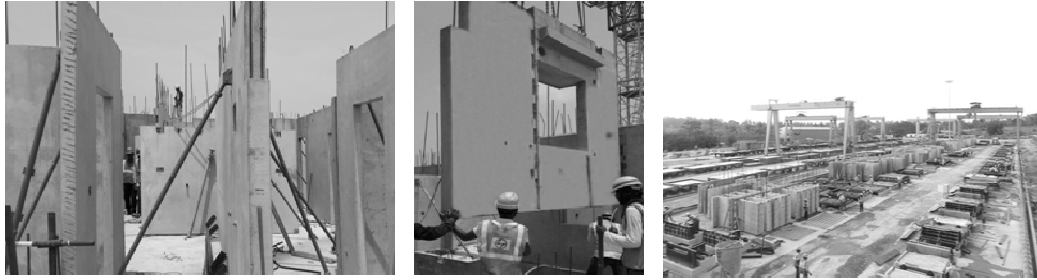
Figure 16: Precast Erection Figure 17: Precast Yard
